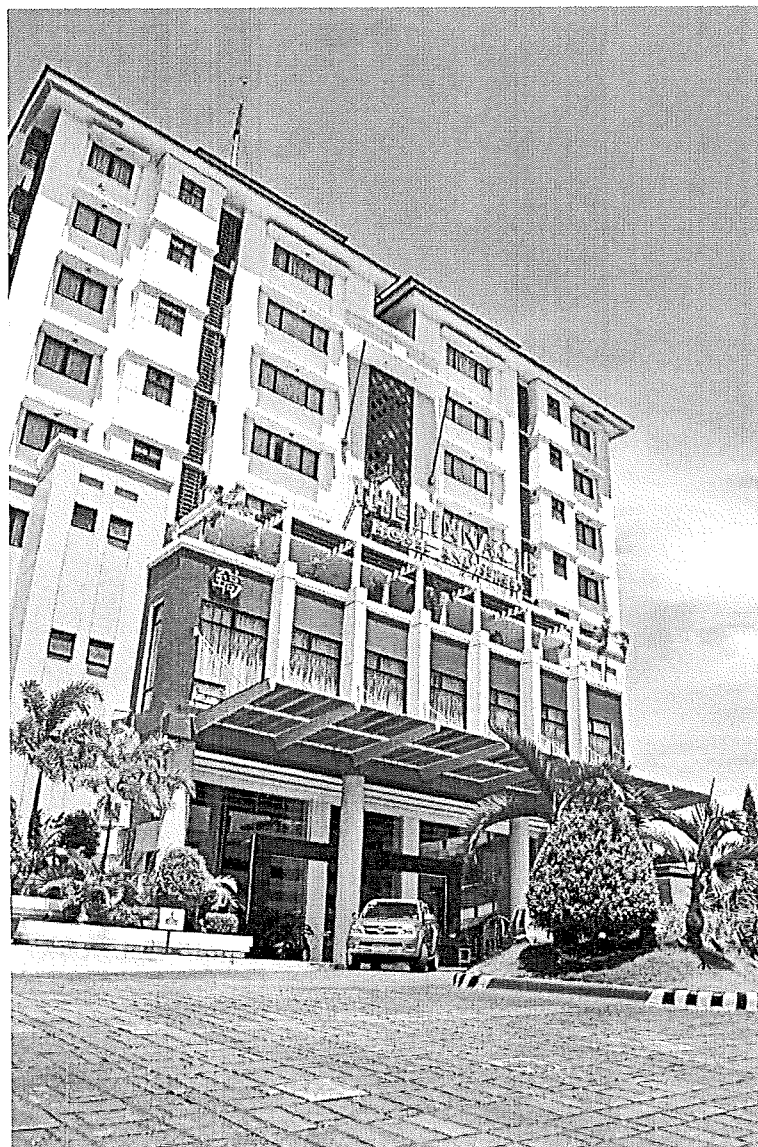
Figure 1. Outside view of Pinnacle Hotel And Suites (Package C) Location: Sta. Ana Ave, Poblacion District, Davao City, 8000 Davao del Sur
